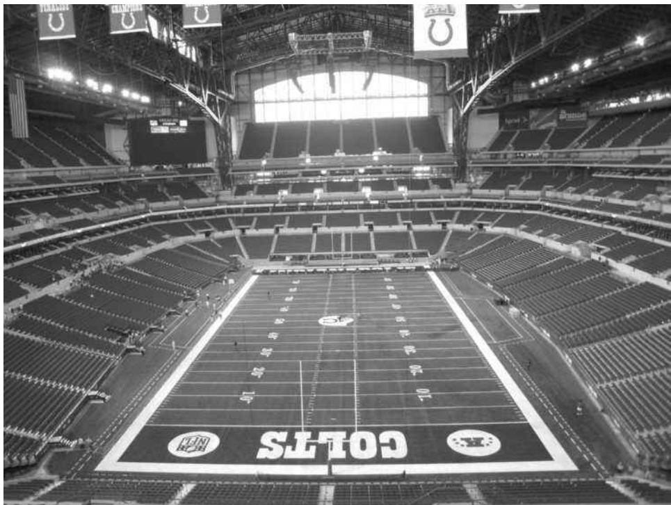
FIG. 14-1 Lucas Oil Stadium in Indianapolis, Indiana
